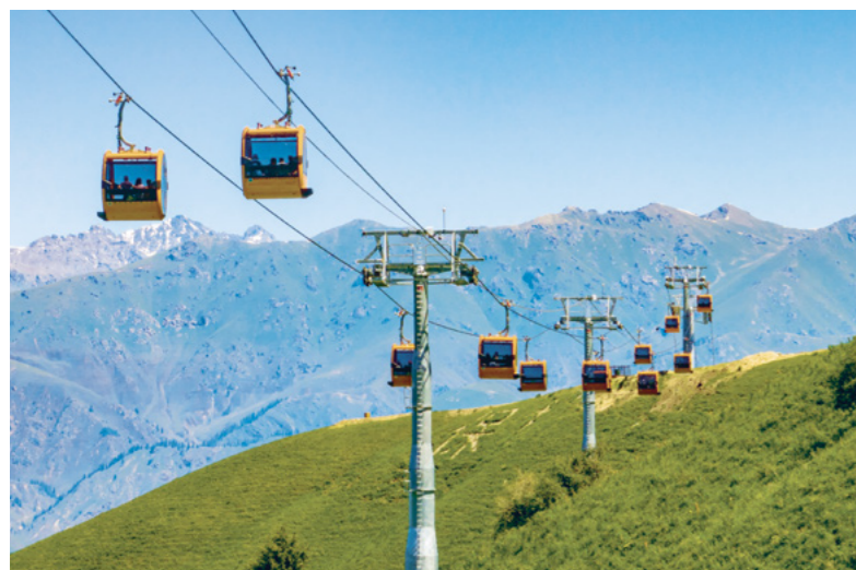
Detachable 8-Seater Gondola Lift | Nalati | China | Design by Studio F. A. Porsche
