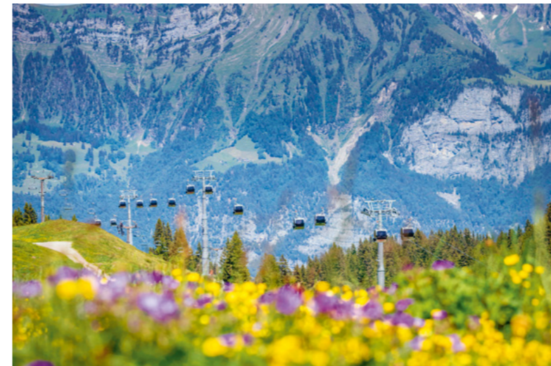
Detachable 8-Seater Gondola Lift | Flumserberg | Switzerland Design by Studio F. A. Porsche
