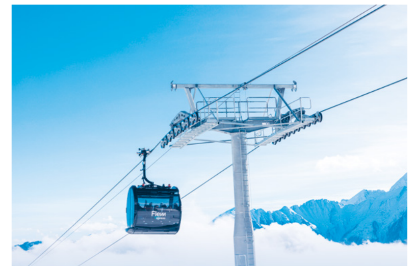
Detachable 10-Seater Gondola Lift | FlemXpress | Flims | Switzerland Design by Studio F. A. Porsche
